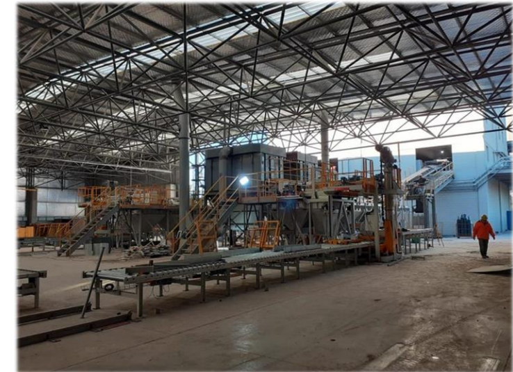
New dispatch centre close to completion
