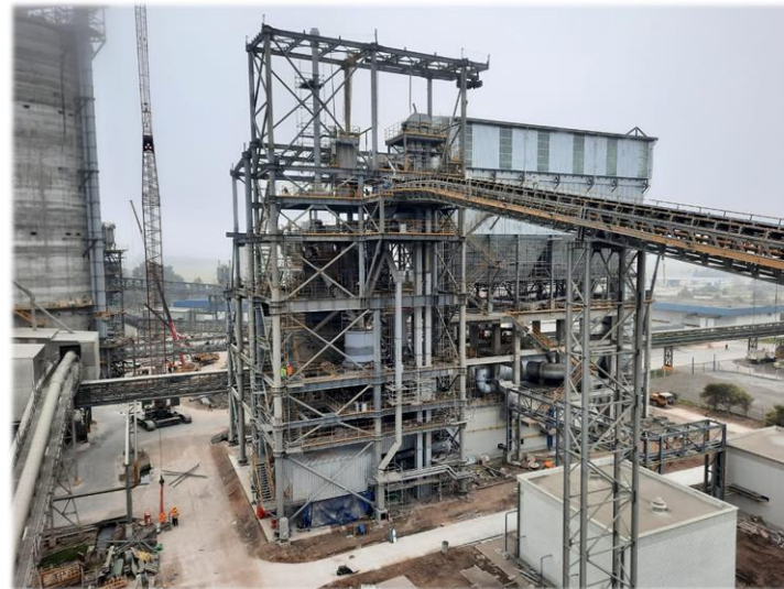
New Cement mill close to completion
