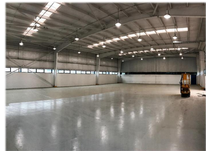
L'Amalí 2: Warehouse expansion
