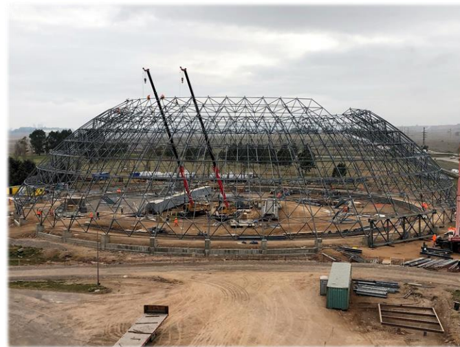
L'Amalí 2: Pre-Homogenization Dome
