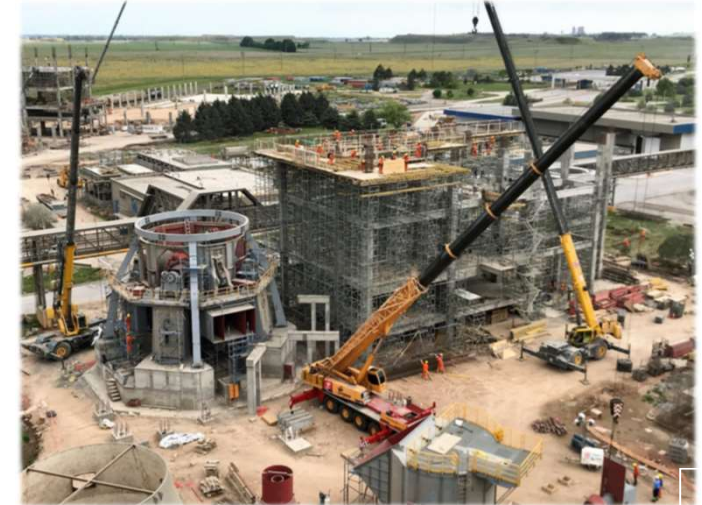
L'Amalí 2: Cement Mill progress
