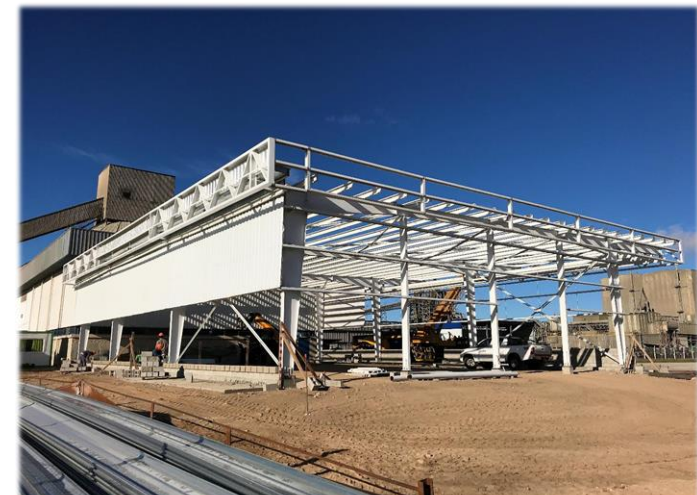
L'Amalí2: Warehouse expansion
